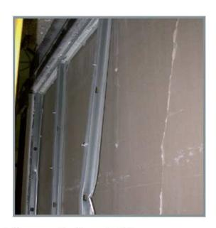
Different levels of damage to Knauf systems, when moving horizontally or vertically up to 27mm
